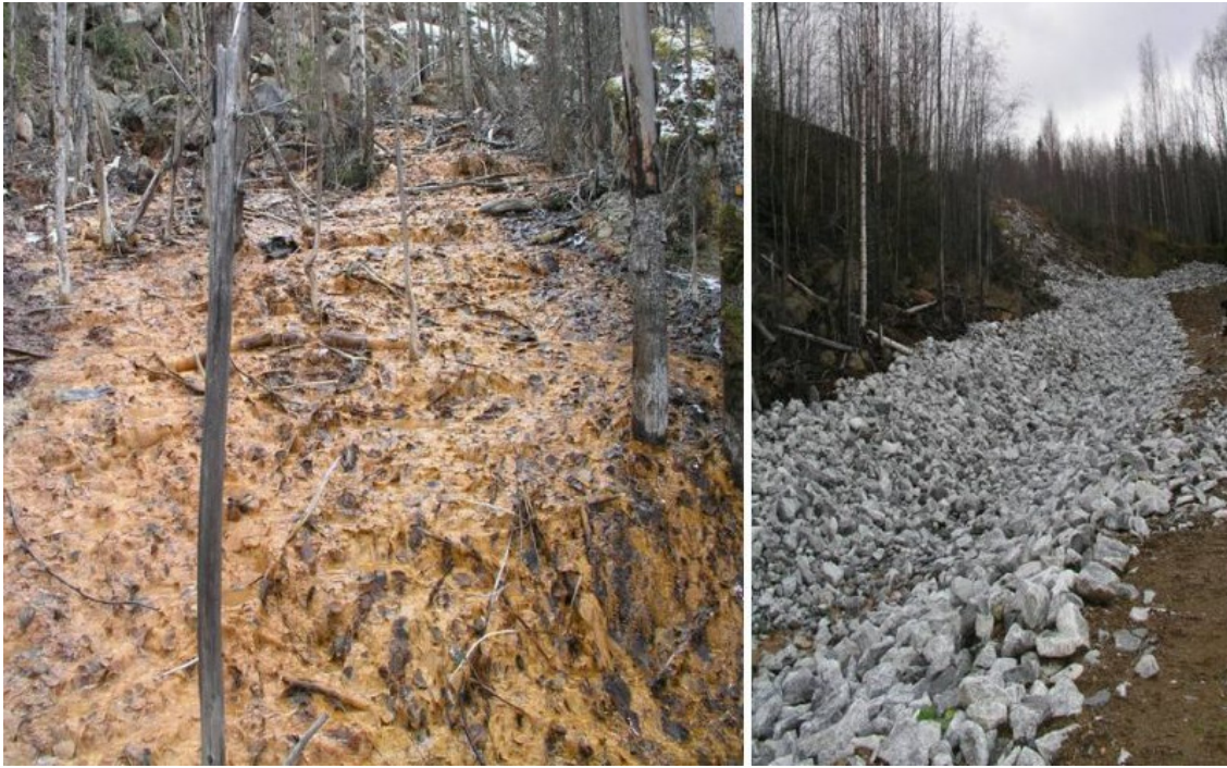
Example of how open limestone channels can be used to mitigate and remediate AMD from seepage areas. This photo was taken at the Luikanlahti copper mine in eastern Finland. Source: Mine Closure
